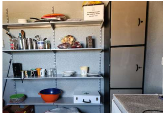
New cupboards and shelving installed in the school kitchen
